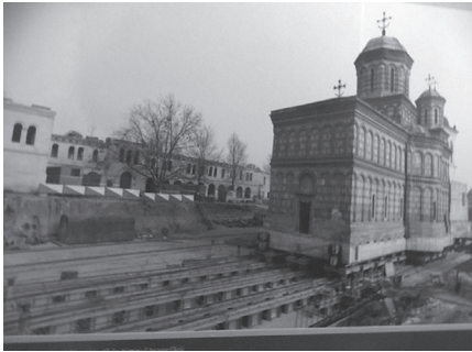
4. Moving a church on railway lines in Ceaucescu's Bucharest
